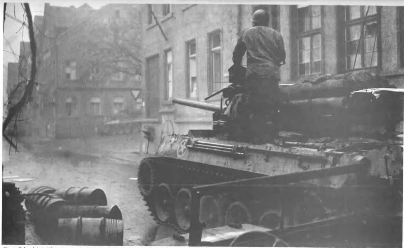
Roadblock! A Third Army Hellcat guards a liberated intersection in a German town while a second tank destroyer, seen in the distance, covers another avenue of approach. Note the spring-equipped tie down for the radio aerial, the gun cleaning rods on the left side of the hull, and the air identification panel covering the top of the box strapped to the back of the turret bustle. An empty carbine rack can be seen above the dashboard of the Peep in the foreground. U.S. Army Photo SC 392730
