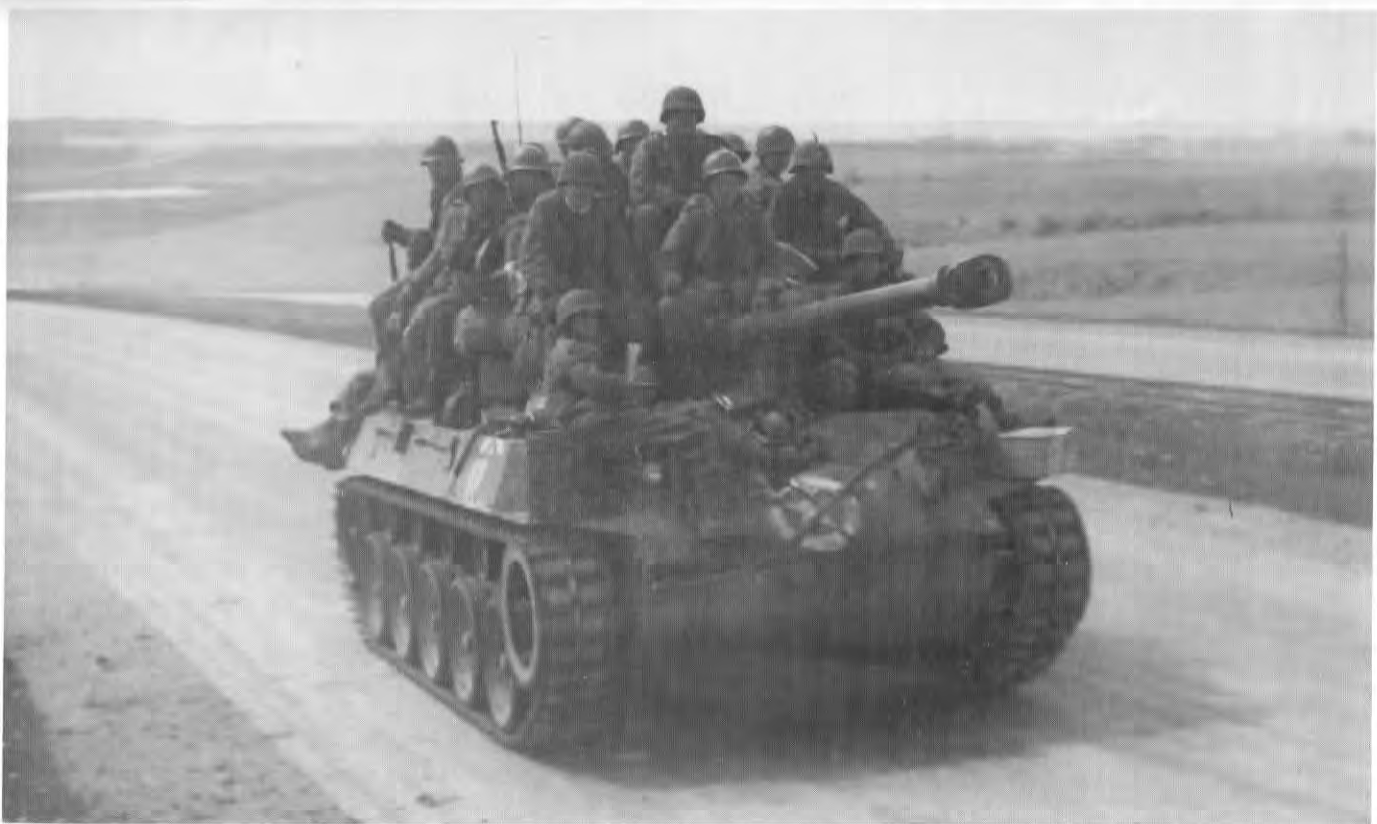
Blitzkrieg American Style! Infantrymen crowd a Hellcat of the 822nd Tank Destroyer Battalion as it speeds along one of Germany's famed autobahns. Such scenes were common place during the rapid advances in the waning weeks of the war. Note the double-barreled muzzle brake in this late model M18 Gun Motor Carriage. US Army Photo SC 206022
