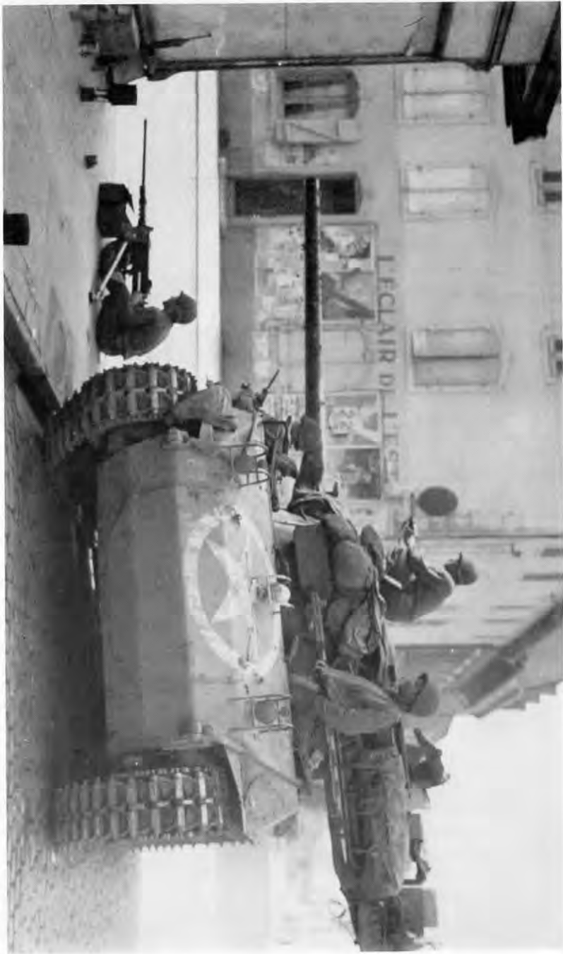
Events down the street cause the crew of this Hellcat to man their guns. The ration boxes and .50 caliber machine gun dismounted from its turret ring-mount indicate that they plan to stay awhile. Although the censor has obliterated the unit markings, details of the siren, headlights and panel allowing access to the transmission are readily visible. US Army Photo SC 194638
