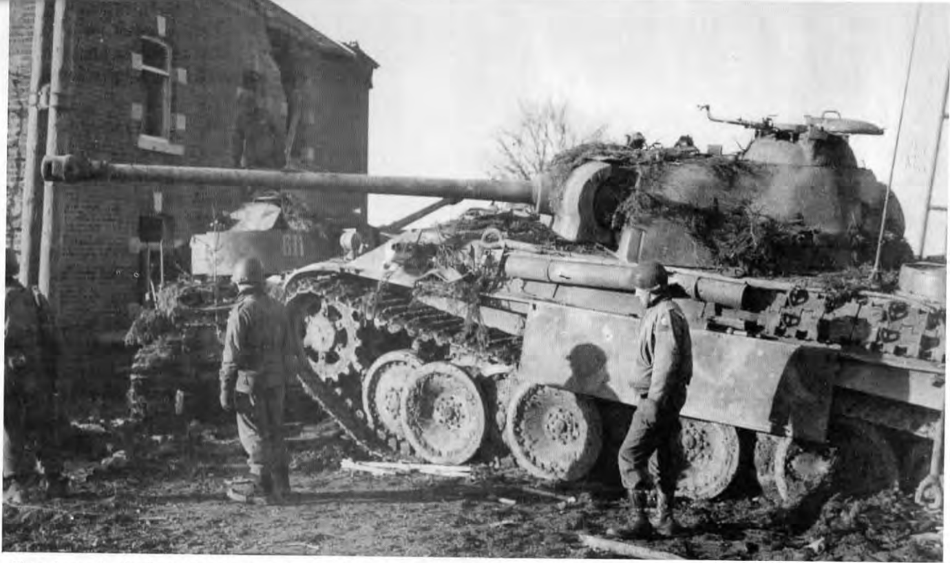
This photo clearly shows the length of the Panther's main gun tube, as well as the clean lines and well-sloped armor of the German tank. Note the destroyed Panzer IV . in the background; both enemy tanks were knocked-out in bitter fighting in Hotten, Belgium, December 26, 1944. U.S. Army Photo SC 197822.
