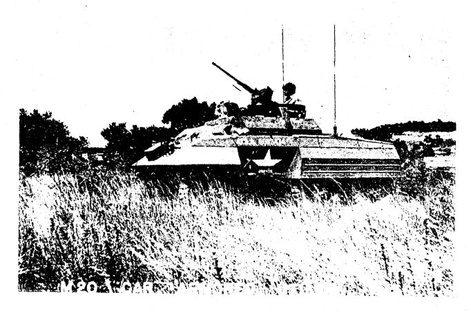
Car, Armored, Utility, M20 (6x6): Vehicle utilizing Light Armored Car M8 chassis was designed to provide a highly mobile armored personnel, cargo carried, and field commander's car. Space is provided to accommodate crews of six, in addition to 506 and 608 radios. Armament consists of one machine gun caliber .50 mounted on a ring mount for anti-aircraft protection, a rocket launcher AT, and individual weapons. Basic armor is same as that of the Light Armored Car M8.
