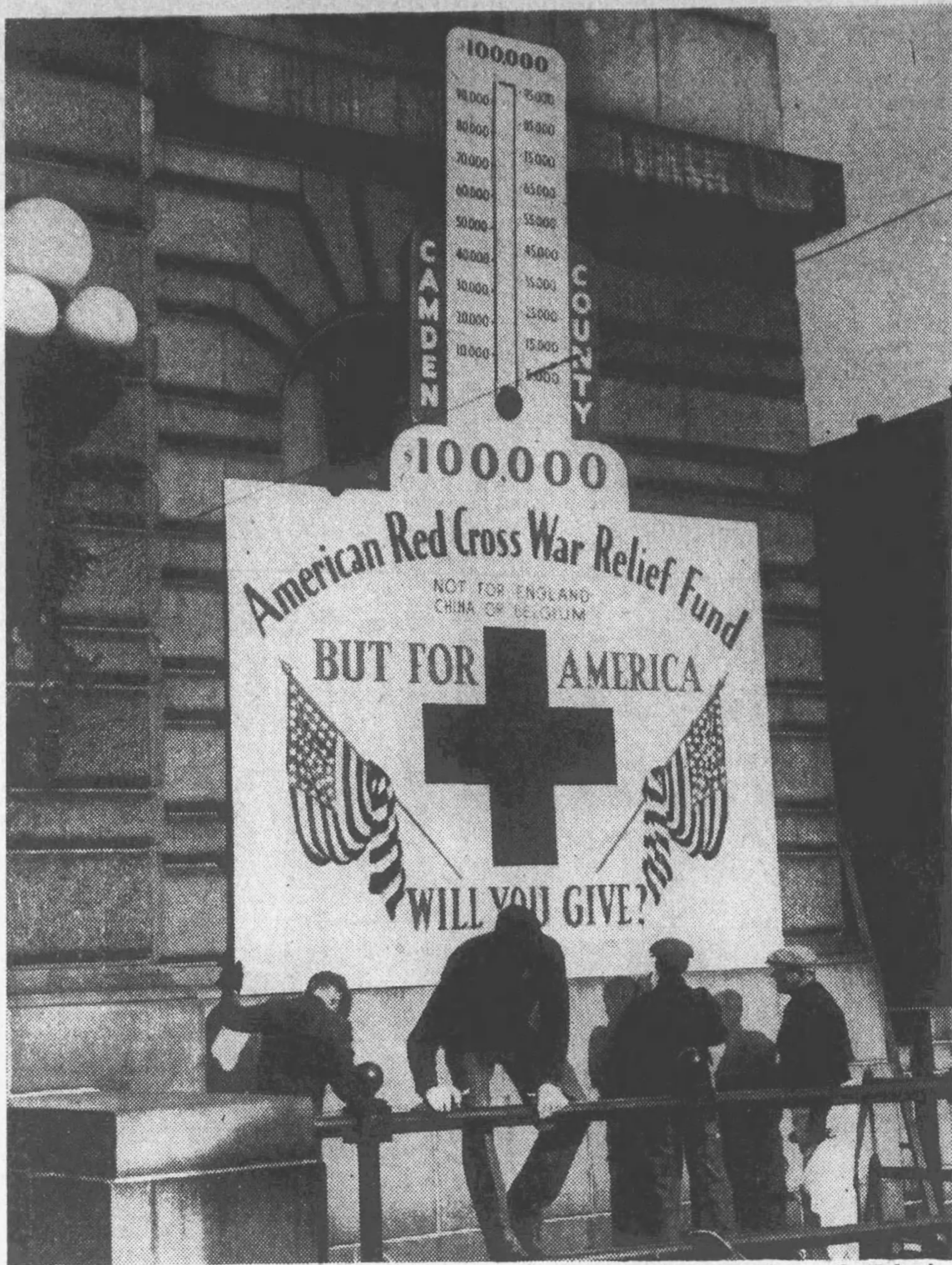
Workmen are shown completing the erection of a giant thermometer and poster on the Federal street side of the old courthouse, signaling the opening of Camden county's drive for $100,000 for the American Red Cross war fund.
