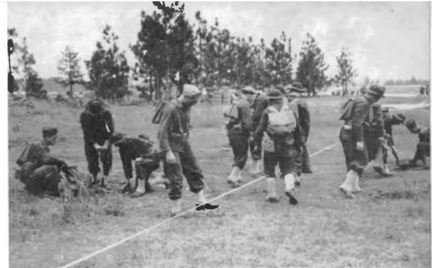
★ Right, reading from top to bottom: Laying hasty anti- tank mines.
