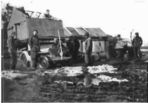
House Moving, Lammersdorf, Germany
