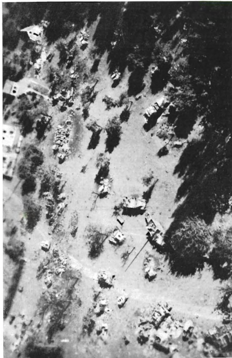
JUST A PORTION OF THE DESTRUCTION AT CHAMBOIS
