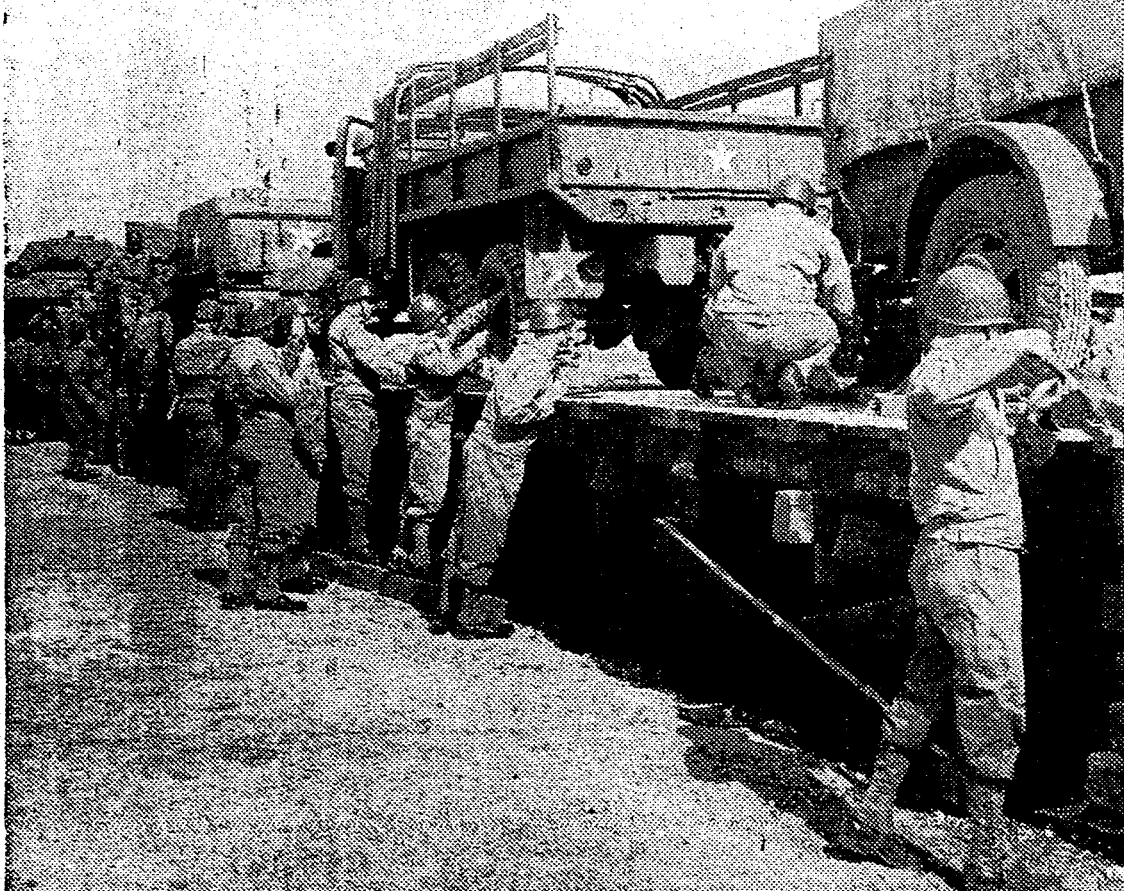
'DRY RUN' RAILWAY —Members of Officer Candidate Class 29 secure vehicles to flat cars of the "Tank Destroyer School Railway" as part of the practical work in the TDS Tactical Department course on vehicle loading and rail movement. See story below.
