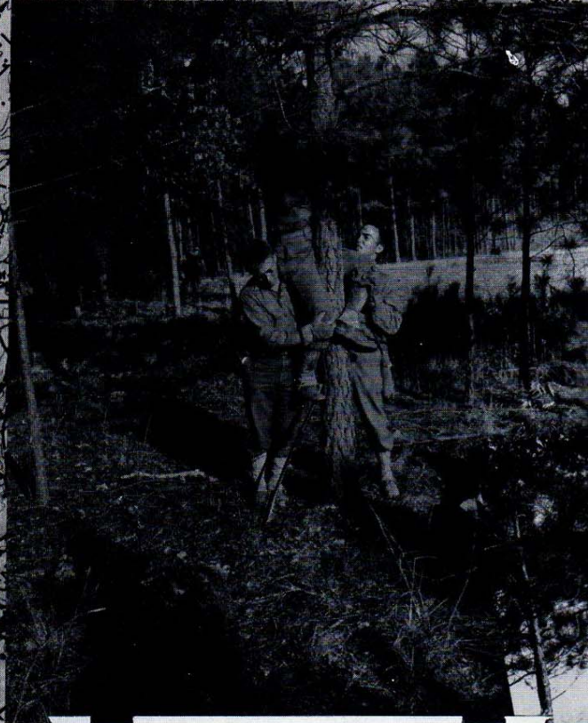
186th F. A. detail laying wire.
